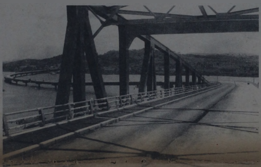
San Juanico Bridge linking Leyte, Samar
