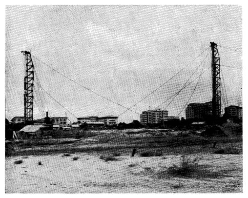
These two Vibro pile drivers are completing the work of driving about 640 concrete piles to support the new home of the American High Commissioner on Dewey Boulevard, which is being constructed by the Marsman Building Corporation. The bottom view shows the completed piles in place. After the piles have been driven a steel and concrete foundation will be built on them.
