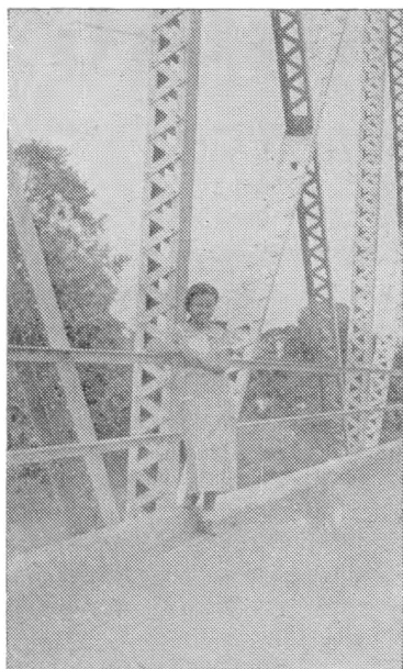
Spanning the Calao River is a bridge the construction of which contributed a great deal to the growth of Santiago. Above is a partial view of the bridge, with Miss Enriqueta Abad, who has on several occasions presided over the town's festivities.
