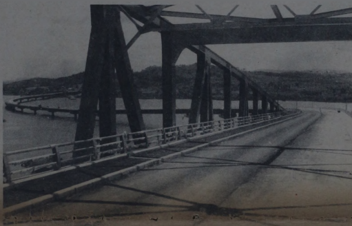
San Juanico Bridge linking Leyte, Samar
