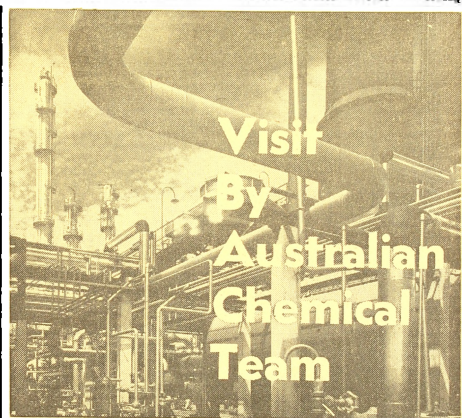
An $111 million olefines plant operated at Botany (Sydney) by ICLANZ Ltd. In the year 1969-70 the Australian chemical industry exported products worth more than $136 million.
