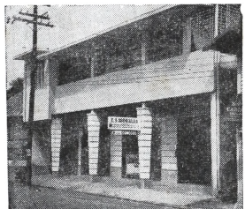
E. S. Morales Company, September 6, 1949. This modest beginning was the INTERNATIONAL HARVESTER dealership after the war destroyed the original building.
