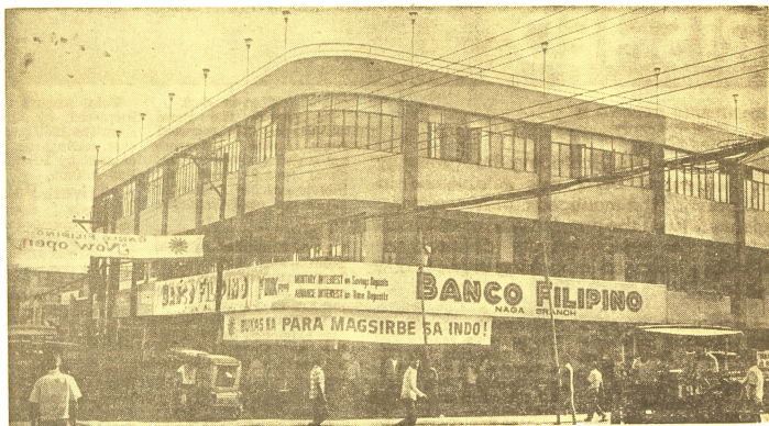
Banco Filipino Provincial Branch
