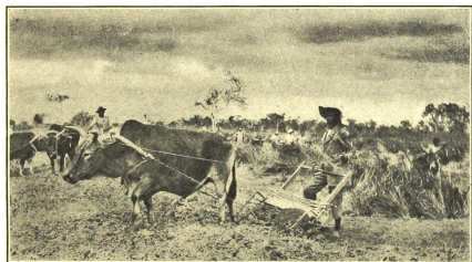
Students grading a road. The rice harrow, or "suyod," is excellent for this purpose.
