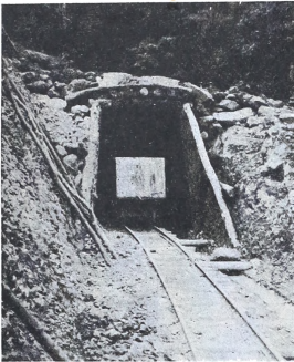
Main tunnel portal cuts ore 266 ft. below surface.
