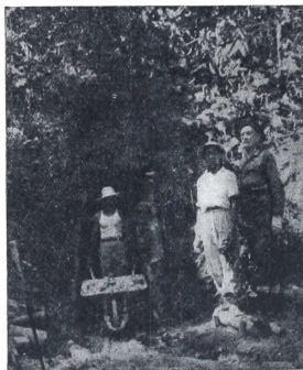
Tunnel 16, Portal and at the side, Lionel D. Hargis with the mine boss.
