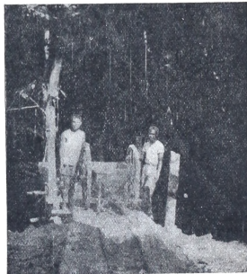
Portal of the Main Tunnel.
