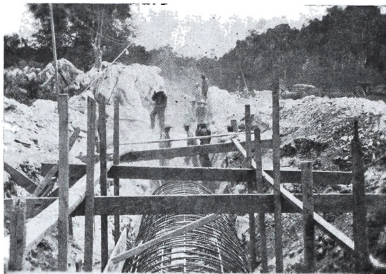
The Ipo-San Juan Aqueduct while under construction.
