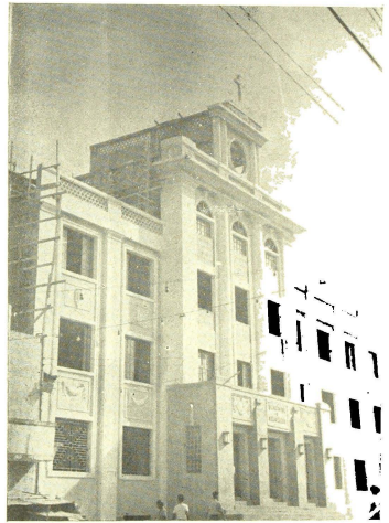
The work completed presents an eye-filling, imposing structure.
