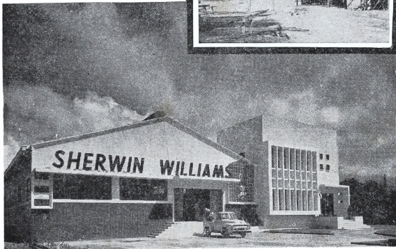
The new Sherwin-Williams building in Makati. It has a 70' rigid steel spin. Structural steel parts were fabricated and erected by A.G.&P.
