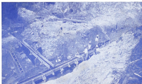
Testing Placer Diggings with Sluices
