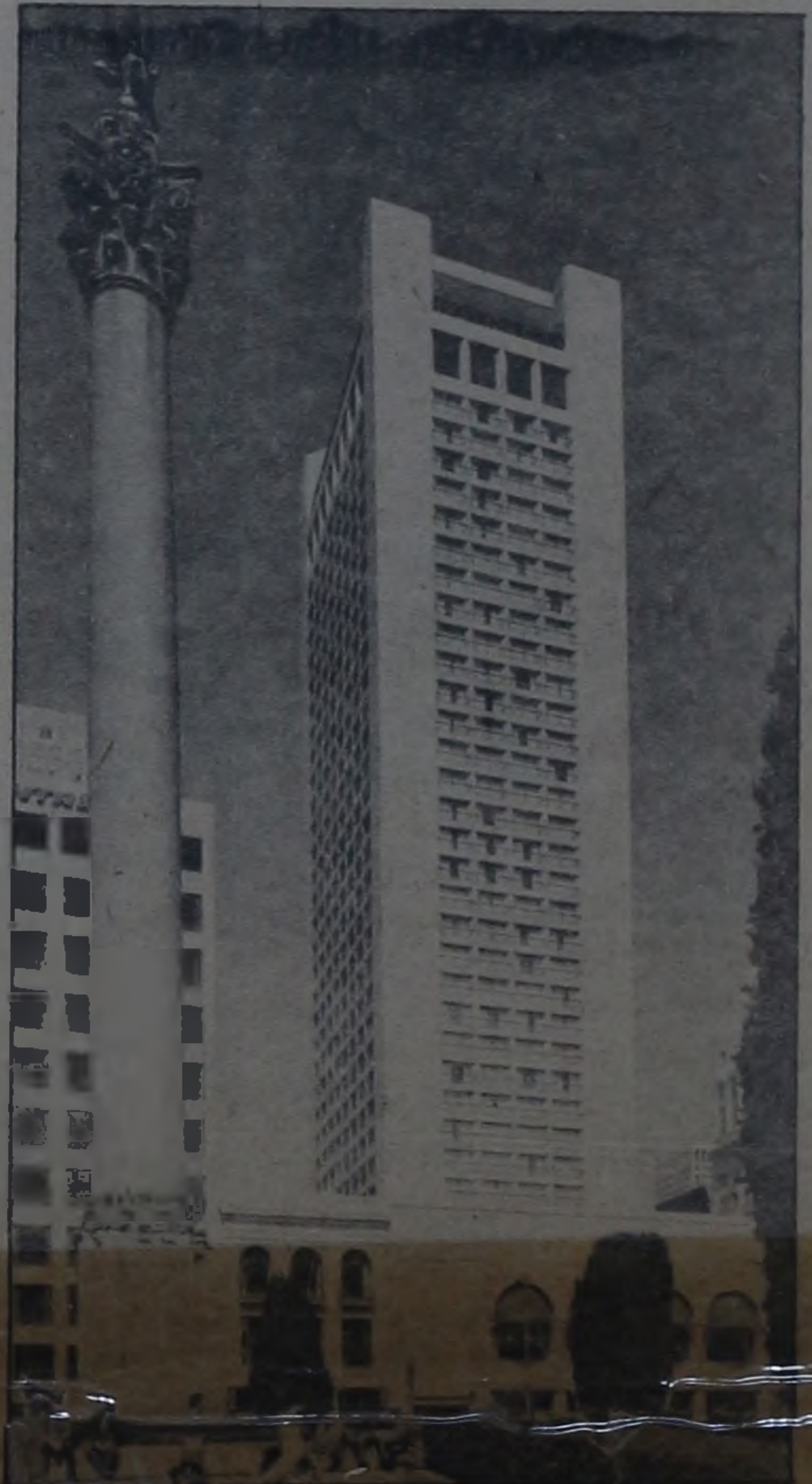
FACADE - Hyatt on Union Square
