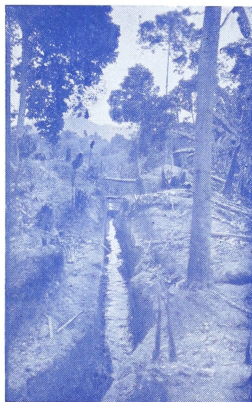
Placer testing ditch 2 kilometers through the claims and down to bedrock
