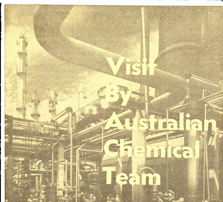
An $111 million olefines plant operated at Botany (Sydney) by ICLANZ Ltd. In the year 1969-70 the Australian chemical industry exported products worth more than $136 million.
