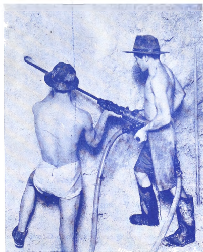
Ingersoll-Rand Jackhammer in use at Benguet Consolidated Mng. Co. Photo by Merl La Voy
