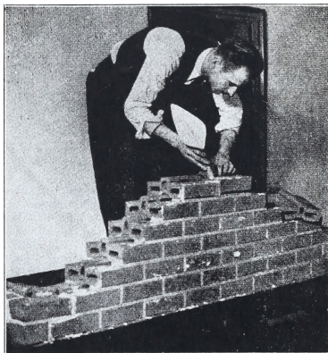
A dry, insulated wall, economical of mortar and speedily laid up, is provided by a new brick unit. Its interlocking joint offers a positive water stop and also makes the unit self-aligning.
