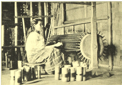
Plate VIII. A cylindrical warping frame.
