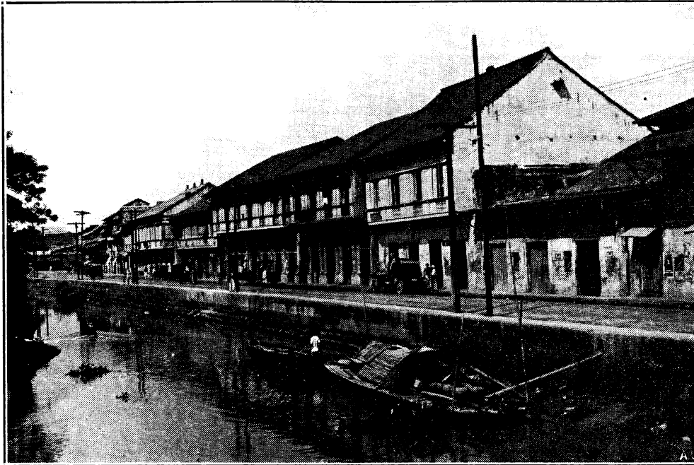
Calle Tetuan: Skirting a Neglected Canal
