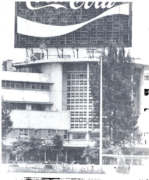
Jai-Alai building on Taft Avenue: Only rivaled by basketball
