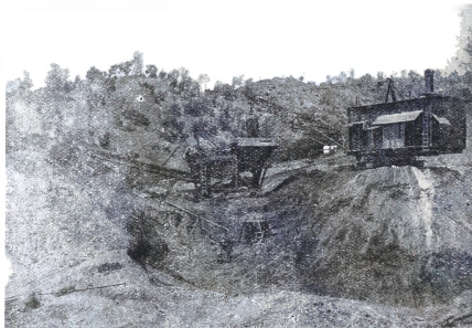
A 60-foot boom carrying a 1½ cubic bucket dumps the gravel into the washing plant. The drag-line excavator makes a complete circle, 120 feet, maximum cut, at each set-up of the machines.
