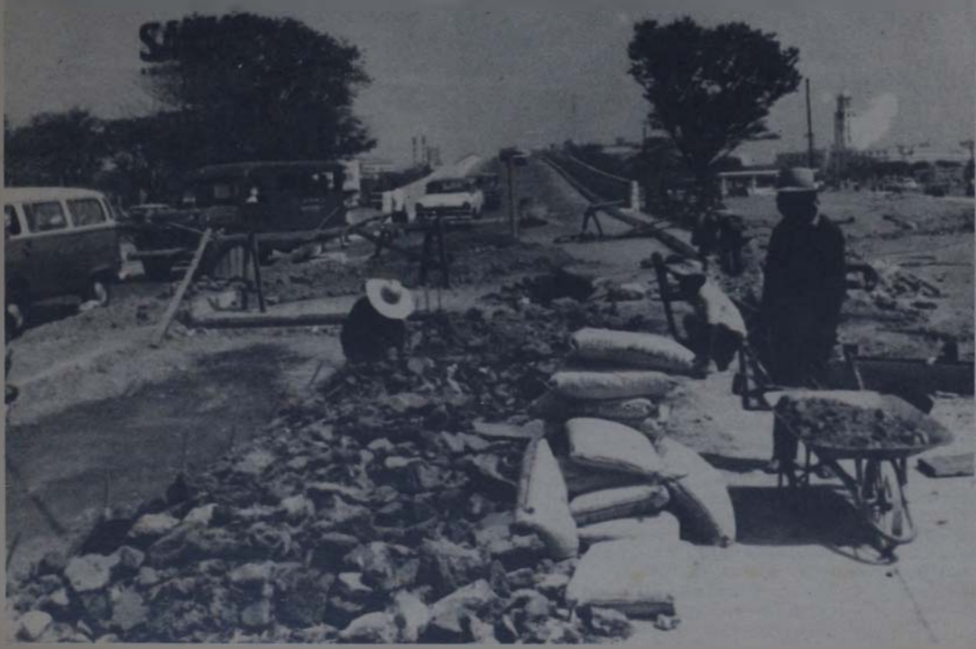
Manila construction project: beating the deadline before the onset of the rainy season.
