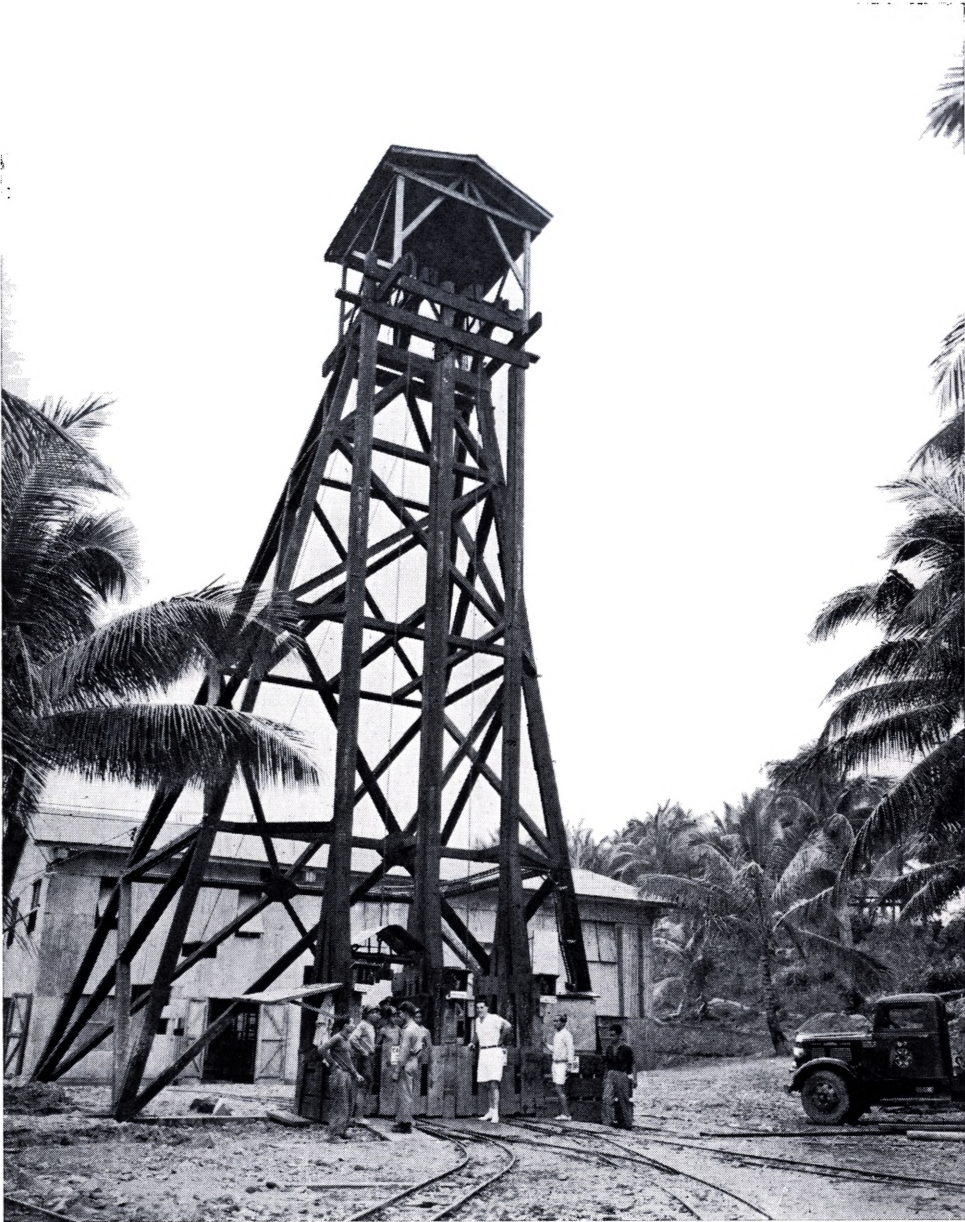
The new headframe at Longos Point, United Paracale Mining Company. Mat Jarvie, who is in charge of operations in this section of the United Paracale mine, is shown at the cage gate with a group of his men.
