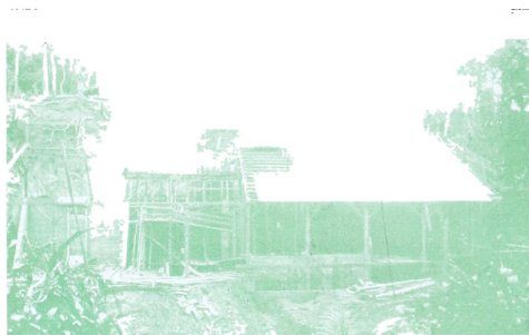
The Tuba mill building.
