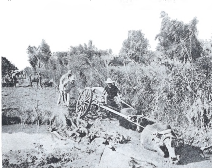
Naic-Indang Road, Cavite, Before Improvement
