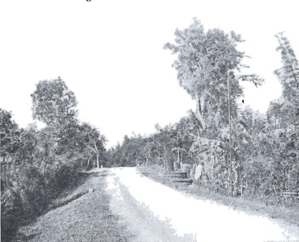
Naic-Indang Road, Cavite, After Improvement
