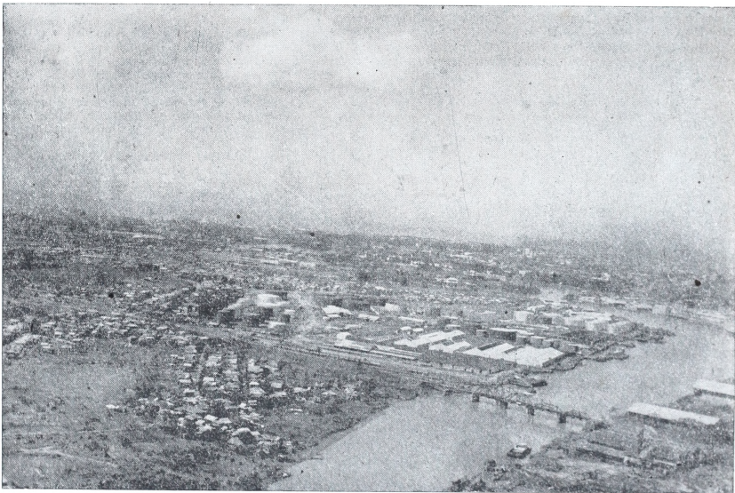
Reproduction of another photograph, taken at 1500 feet, showing the Pandacan Oil Terminal within a loop of the Pasig River.
