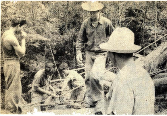
Preparation of rigging for the Gravity Slack line system of hauling logs.
