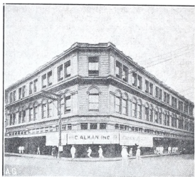
Alkan Building, Escolta: Fourth Story Added Since Picture Was Taken
