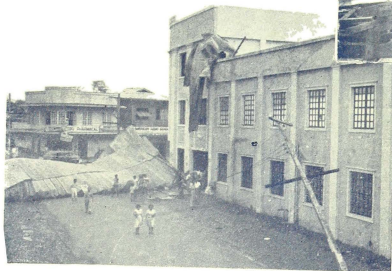
The USC Science Bldg. unroofed by a 100 miles-per-hour wind
