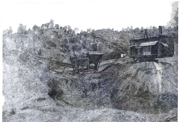
A 60-foot boom carrying a 1½ cubic bucket dumps the gravel into the washing plant. The drag-line excavator makes a complete circle, 120 feet, maximum cut, at each set-up of the machines.
