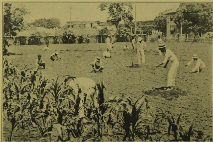
Preparing a school garden, Manila.
