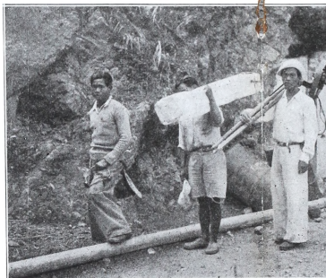
On the march. A crew of Developments, Inc., ready to move to a new set-up, a protection against the weather, and it takes five men to
