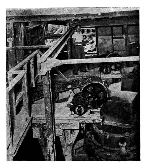
The first step in a cyanide operation. Ore going to the primary crushers, from which it will go to the ball mills to be ground in a cyanide solution.
