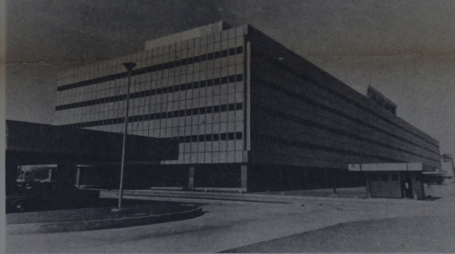
The new Central Bank building: symbol of monetary stability.
