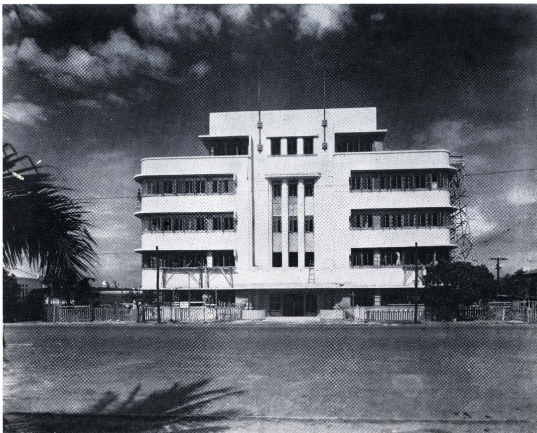
The new Marsman Building as it appears from the Manila Bay side.
