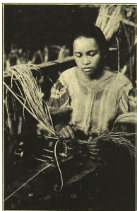
Making rattan splits of uniform thickness.
