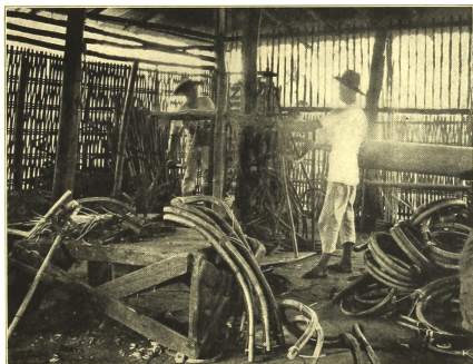
Forcing the rattan onto the V-shaped form.
