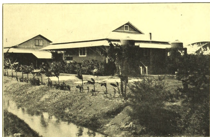
Houses constructed partly by pupils from Haiti Trade School, showing proper use of foliage for screening purposes.
