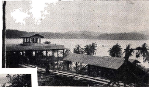
The sample mill is nearly finished.
