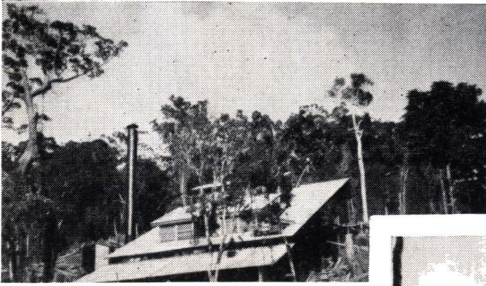
The main smelter building and the smelter stack.
