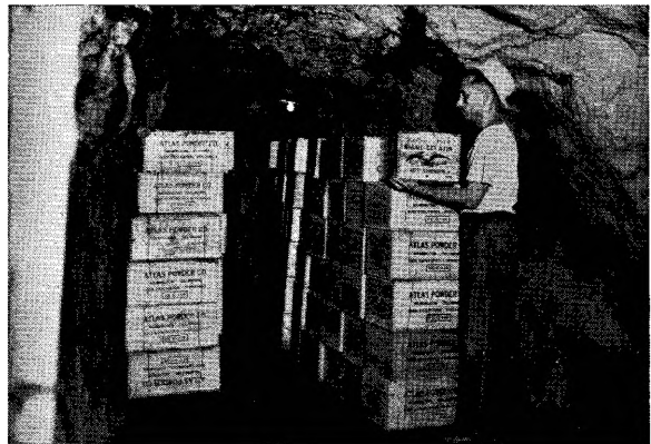
Storing dynamite underground at United Paracale.
