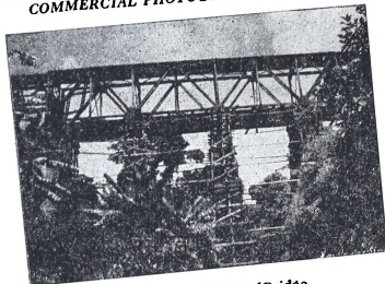
Manila Railroad Bridge
