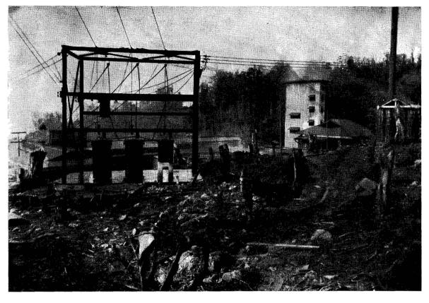
The new Cottrell plant at the Philippine Smelting Company's operation in Mambulao. By the use of this unit, the smoke nuisance will be practically eliminated.
