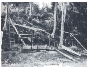
Longyear Diamond drill at work at Malaguit.
