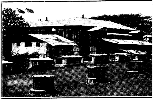
The old San Juan reservoir which figures in the story concluded below has become antiquated, with the development of Manila's modern water system, but remains of peculiar historical interest.—The grilles cap the ventilators.—The large building was, in earlier years, the offices of the water administration.
